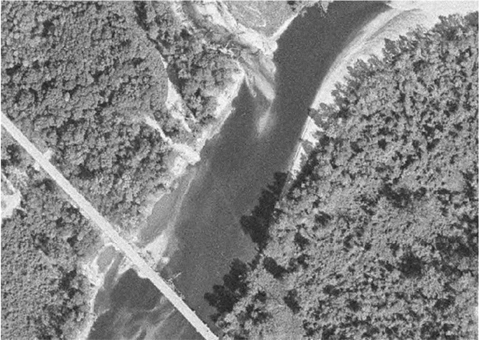
1993: Sand deposition out of sand mine and at old SR 4 bridge pier. Normal sand deposition is not on outside curve of river.
