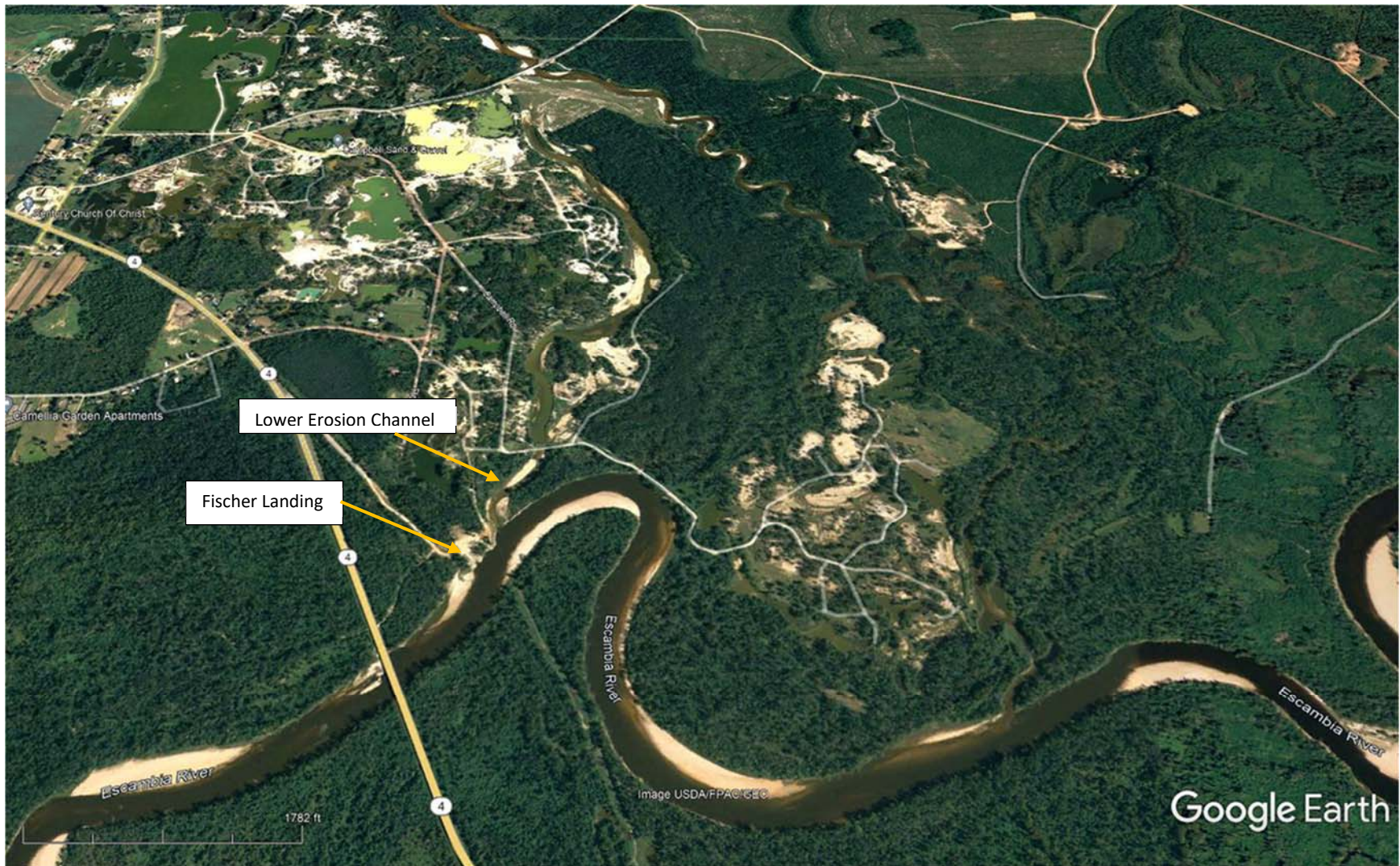
November 2007: Sediment from the lower portion of the Erosion Channel has accumulated at the SR 4 bridge rubble. Fischer Landing boat ramp is not blocked, but the accumulation of sediment indicates that there is an effect on currents in the area.
