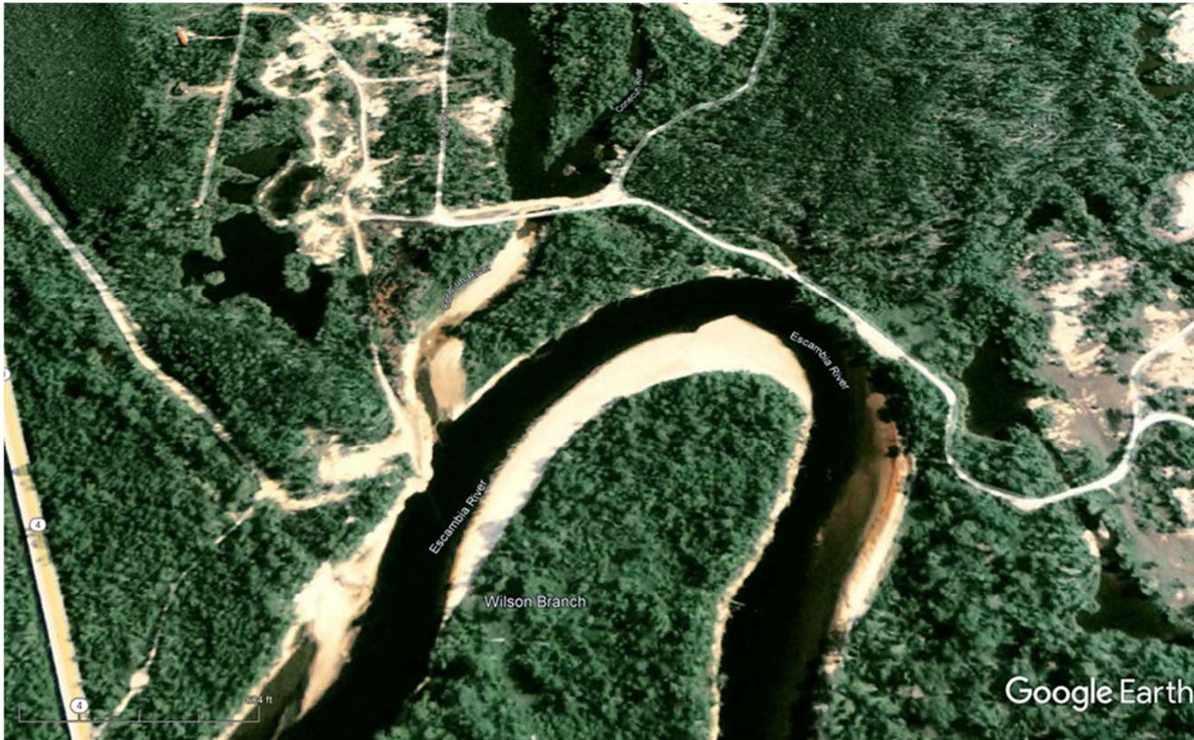
June 2006: Erosion Channel has been blocked by a dam upstream of Flossie Road. A dam is also in place at the eastern Flossie Road bridge. Sediment still impacting Fischer Landing from below the new dam. Bridge pier rubble presents a location for sediment deposition to extend up river to Fischer Landing.
