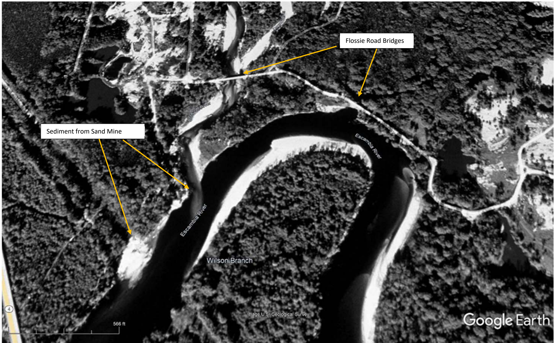
November 1999: Closeup of Fischer Landing location. Sand from western mine location has created a sub-surface sand bar at the outfall location. Sand buildup in the vicinity (upstream and downstream) of the bridge pier rubble indicate that the structure has some effect on the deposition of sediment load.
